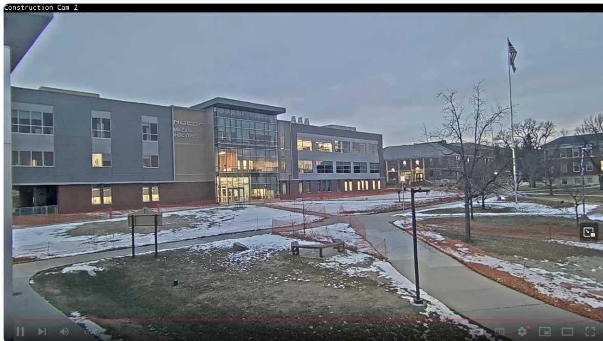
A screen capture of the Nucor Mineral Industries construction camera on December 18 th .
