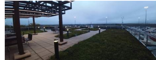
Rapid City Regional and SD Mines green roof project.
